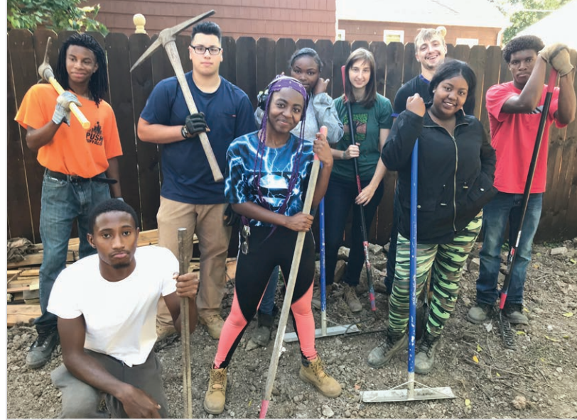
PUSH Blue Environmental Stewardship trainees learning how to install a rain garden.
