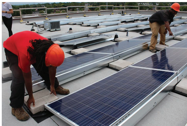
Hiring Hall workers installing solar panels on the roof of School 77.
