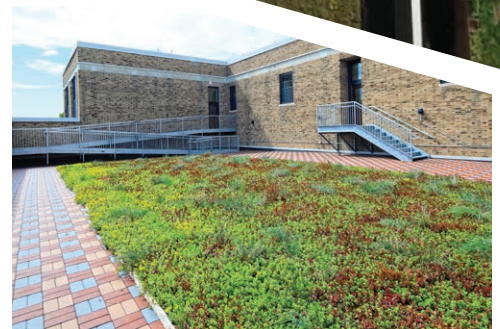
Green roof and outdoor space for School 77 senior residents.
