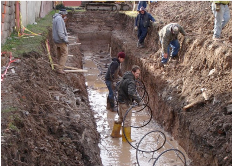
Installing the geo-thermal system at the NetZero house in the GDZ.
