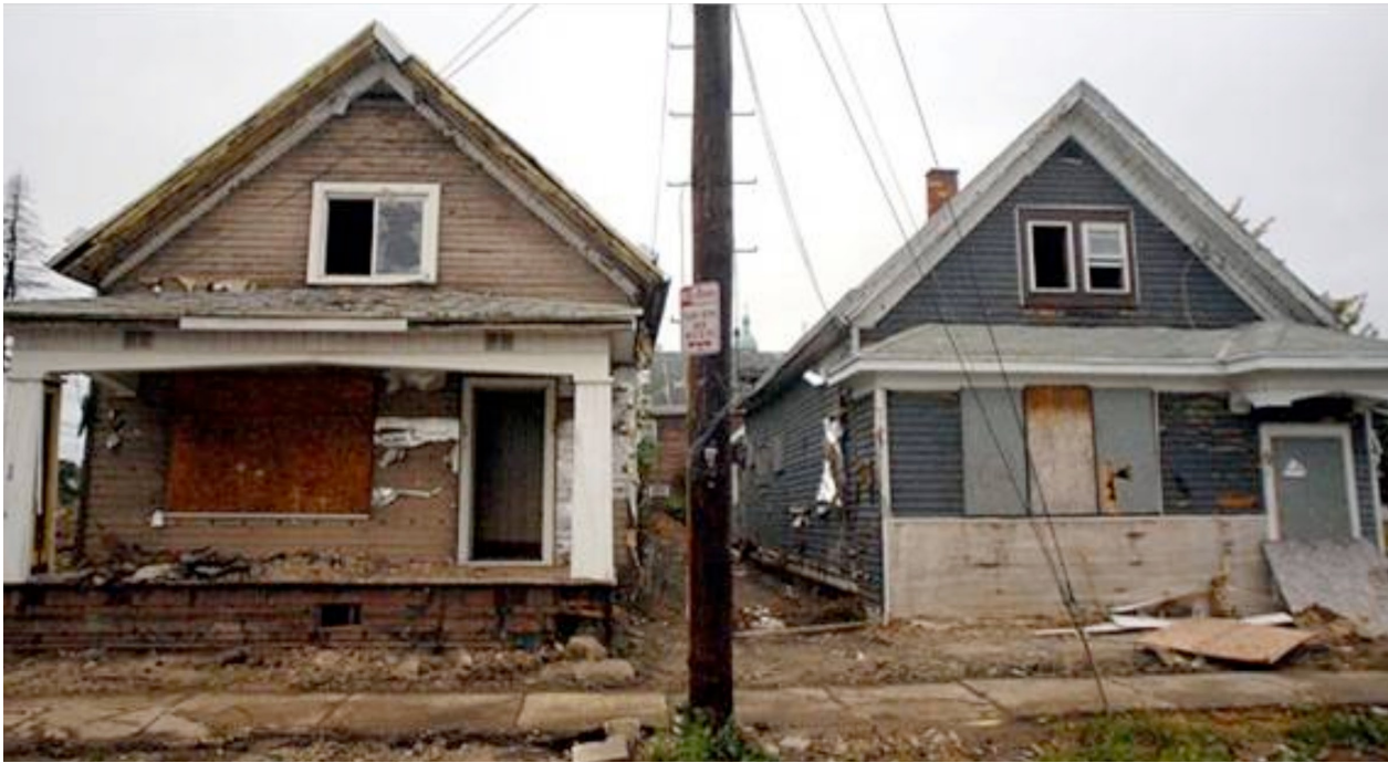
Two of more than 15,000 vacant properties in Buffalo.
