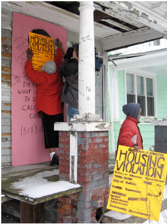
A PUSH member issues a “violation” to state housing authorities for neglecting one of 1,499 vacant properties under state control in Buffalo.
